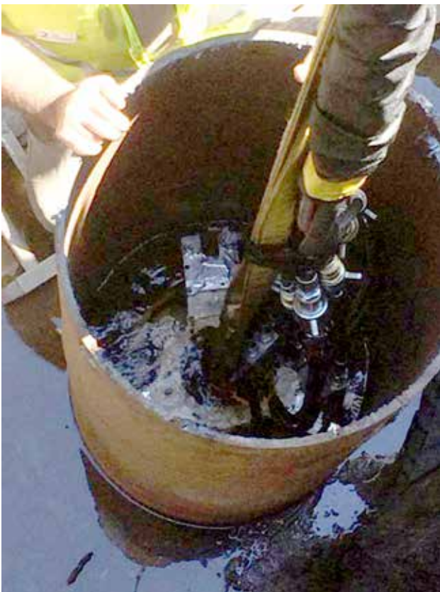
Bridge Piling Cutting
